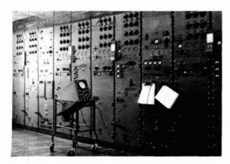
fig. 4. The diversity receivers used by RCA Communications, Inc., Riverhead, Long Island, New York. Notice the clipboards in the center; these held the receiver log. The log clipped at the top, in the usual way, indicates that receiver is in use. The log held by the corner indicates that that receiver is on standby. The index file on each receiver gives dial settings for commonly used frequencies. (Photo courtesy Robert McGraw, W2LYH, and Harlod Moore.)
