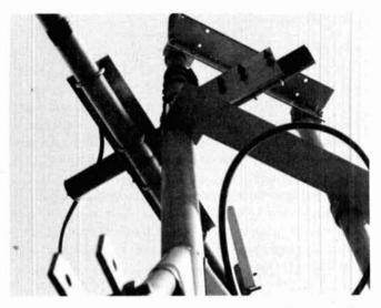
Two angle brackets are used to hold the auxiliary mast in place. One is attached above the 40-meter tilt assembly; the other is connected below.
