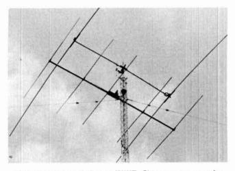
The antenna installation at W1XT. Shown are a two-element, 40-meter Yagi and an understacked five-element, 10meter Yagi.
