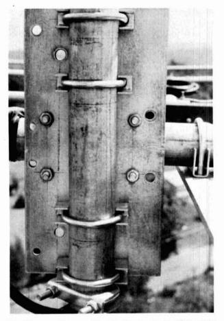
The 10-meter tilt assembly attaches to the auxiliary mast with four muffler clamps. Note the clamp at the very bottom of the mast. It is needed to keep the tilt assembly from slipping off the auxiliary mast and is an absolute requirement.
