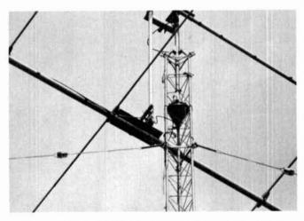
The guy-wire torsion bracket is mounted just above the bottom rung of the tower top section. The 10-meter antenna rotates just above the top set of guys. An empty torsion assembly at the top of the tower is available for an additional set of guy cables if they should be necessary.
