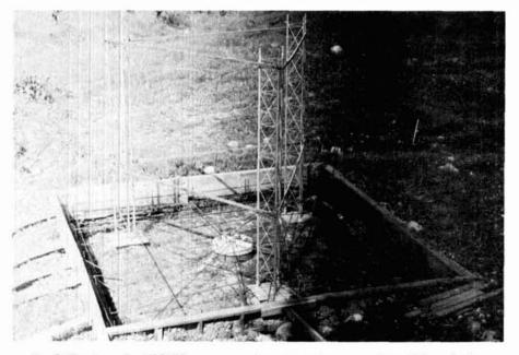
fig. 3. The base for K6QXY's new moonbounce antenna consists of three lattice towers arranged in a triangle. The first sections are up in the photo. The towers will go up to about 80 feet (24.4. meters), tied together every 10 feet (3 meters). Twenty-three cubic yards (17.6 cubic meters) of concrete will be poured into the base.
