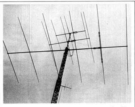
fig. 5. July, 1980. The high-power antenna farm of a prominent East Coast DXer before the winter storms hit. The self-supporting crankup tower held stacked 20-, 15-, and 10-meter arrays, a heavy-duty rotator, and a side mounted 2meter beam. All worked well until.....
