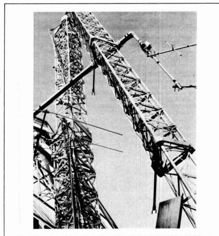
fig. 6. The winter storms hit, and the tower fractured at mid-joint. Luckily, no one was injured when all of this metel tumbled down from the sky. Is your antenna designed to stay up?
