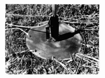
fig. 2. Basic ground system under each radiator, consisting of copper disk and No. 16 insulated ac house wire.
