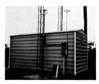
fig. 10. Coax enters building through a weather-proof box. The anemometer is made from a DC motor and recycled air freshener containers.
