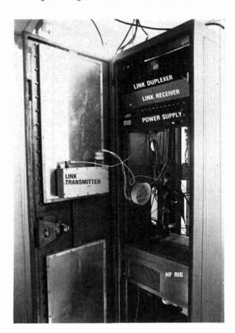
fig. 5. Rear view of cabinet illustrates placement of link components.
