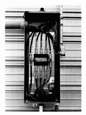
fig. 9. Coax passes through lightning arrestors before entering building.
