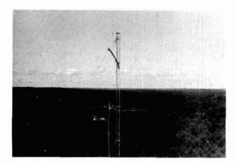
Ground and aerial views of two element 80m delta loop array supported by 46' boom at 115'.
